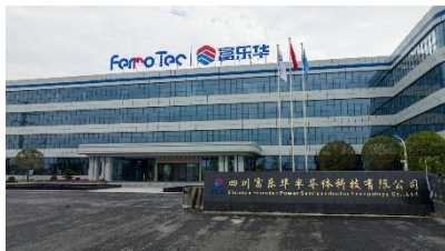
Neijiang Factory (Sichuan, China)
